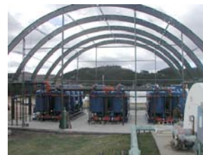
Figure 3: Yardney sand filters replace Baker sand filters.
